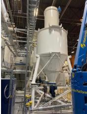
AES was tasked with taking the pre-designed mechanical process of storing the chalk powder in a giant hopper and moving it using
